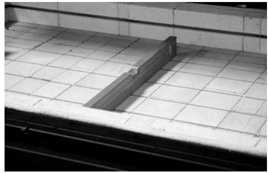
FIGURE 2: CHECKING THE KILN FLOOR WITH A LEVEL.
